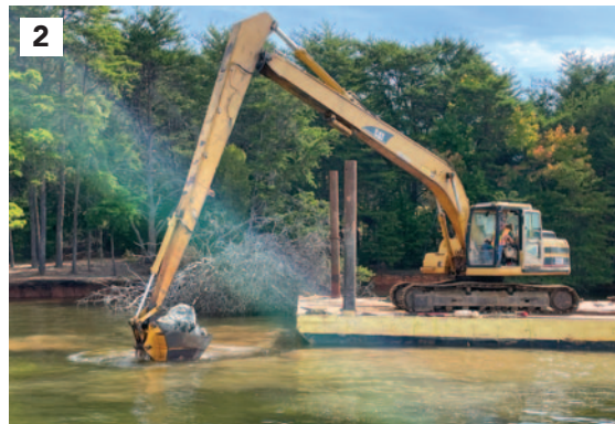
1 and 2. A LARGE BARGE AND CRANE LIFTED AND PLACED 18 LOADS OF ROCK FOR THE ARTIFICIAL REEF.
